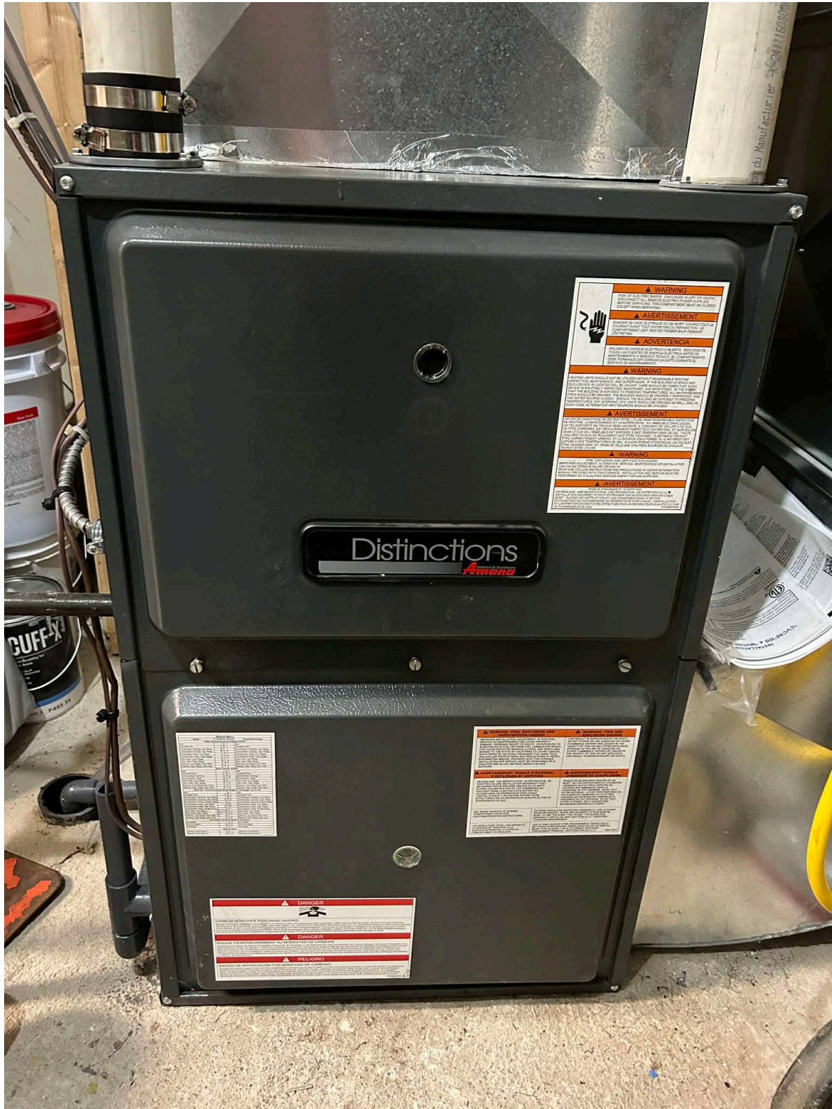
Furnace installed last year (Amana by Goodman, model number GMVC961005CN)
